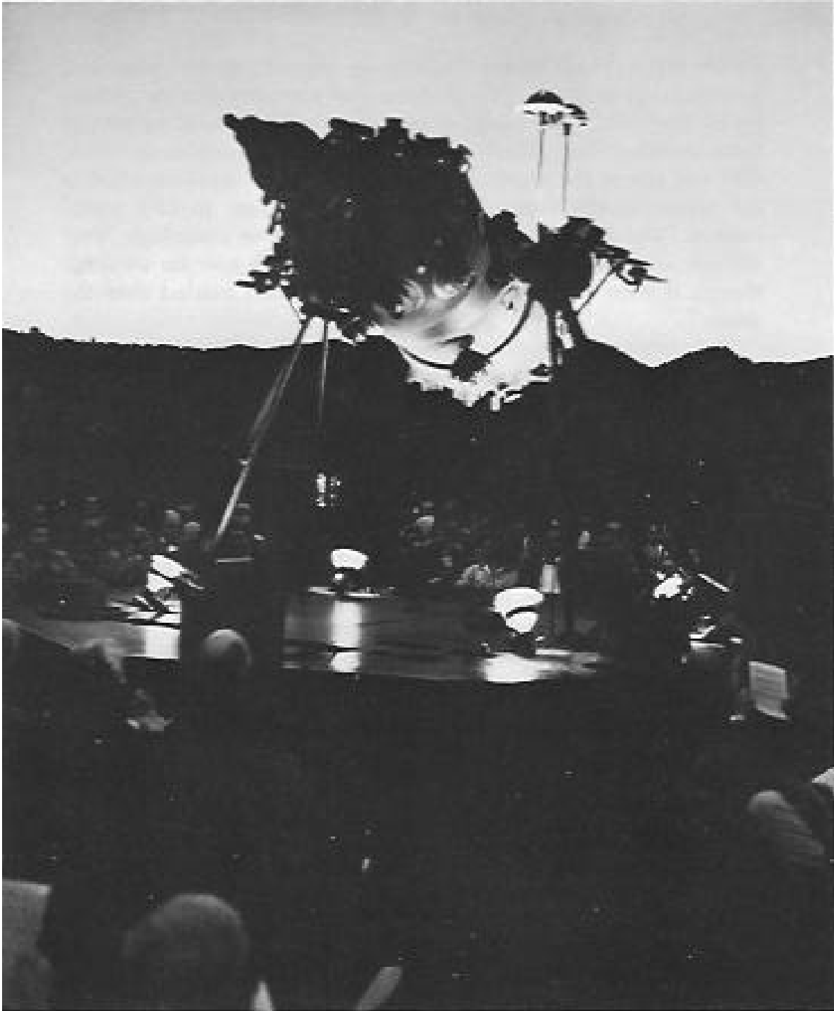
Planetarium projector shown equipped with two interference-pattern projectors ( top right ) for Vortex Concerts.
