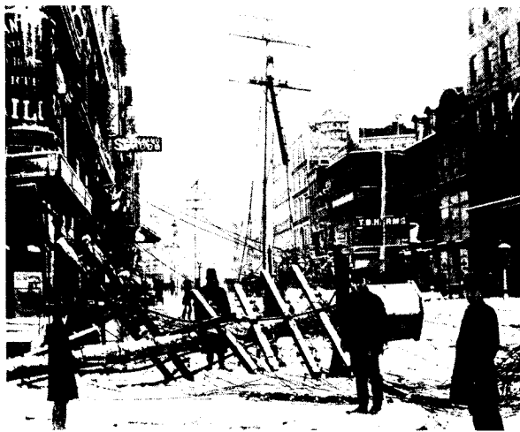
This photograph was taken after the Great Blizzard of 1888, at the corner of Broadway and Twelfth Street. A law had been passed in 1884 requiring all telegraph, telephone, and electric wires to be removed from the streets; the first underground conduits were laid in 1886. The blizzard helped speed the process of cable-laying.
